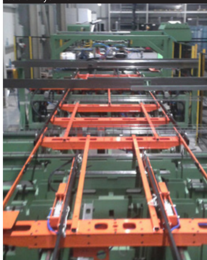
Cable trays line
